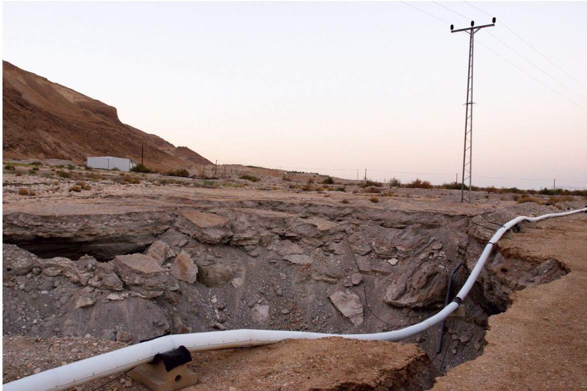
Damage caused by a sinkhole near the Dead Sea, as seen in Yara Saqfahait's research project and publication Subterranean Cavities , 2017, image courtesy of Alamy ( www.alamy.com )
